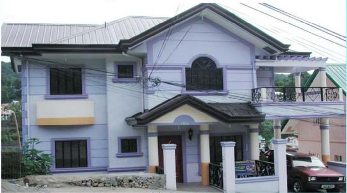
House Built At Woodsgate Compound, Camp 7, Baguio City
